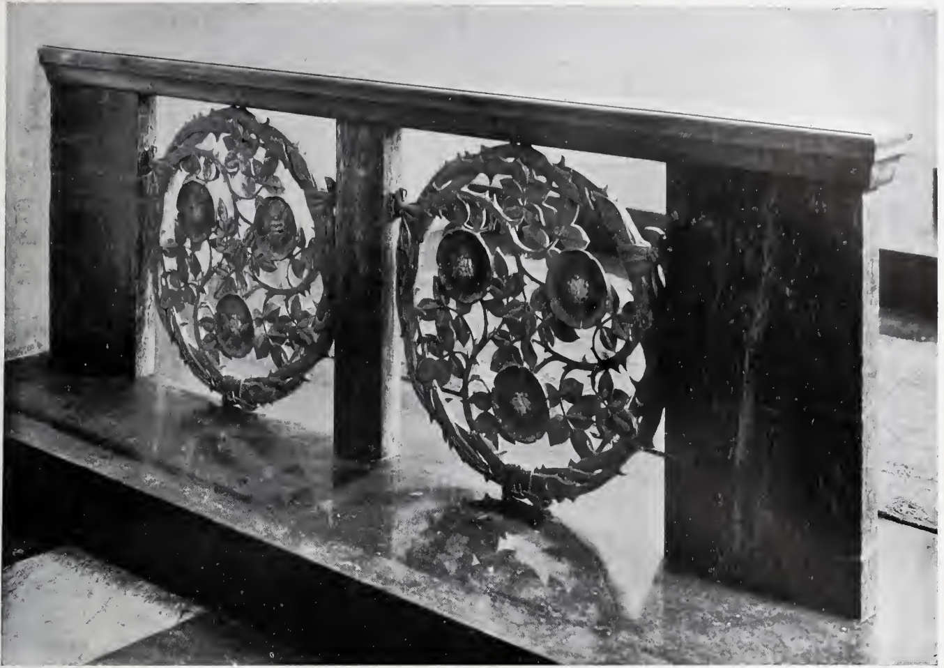
Altar Rail : subject, the Glorified Crown of Thorns. Rail, oxidised grey copper panels in brass uprights, dark Irish green marble; step, dark grey fossil marble.
